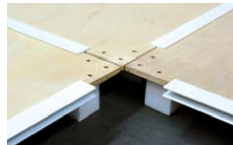
Floor and dynamic foam mounts.
